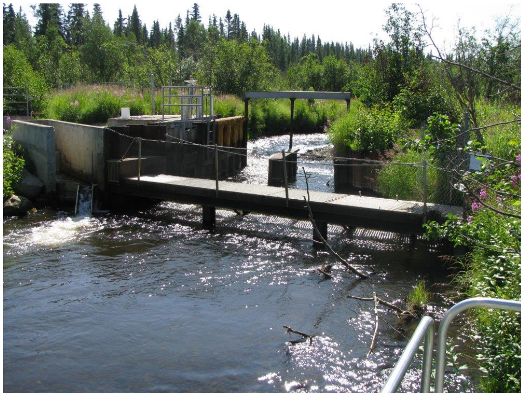
Figure 1. Crooked Creek Chinook salmon weir and fish ladder.
